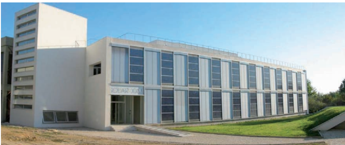
SolarXXI building, showing a 100 m 2 PV façade
