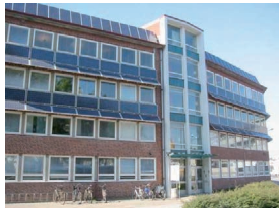
Example of fixed sunscreens over the windows. Malmö Stadsfastigheter - Sweden
