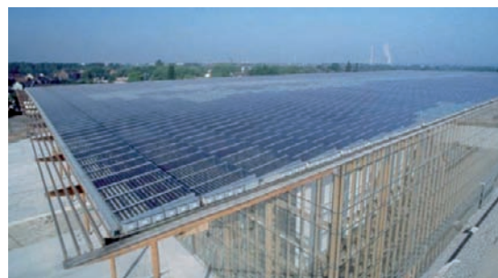
Academy Mont-Cenis, Herne. 10,000 sq m OPTISOL® single glassed overhead and within the vertical façade.
