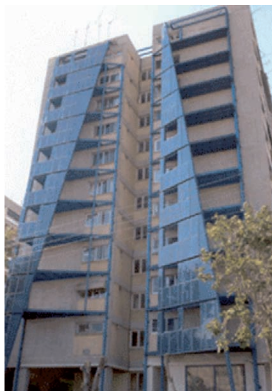
Integration of PV in multifamily dwellings (Tavros, Athens) (by SOURSOS). Integration into façade.
