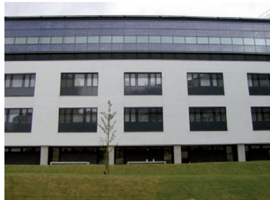
Roof installation in ZICER Building, University of East Anglia. Semi-transparent PV modules
