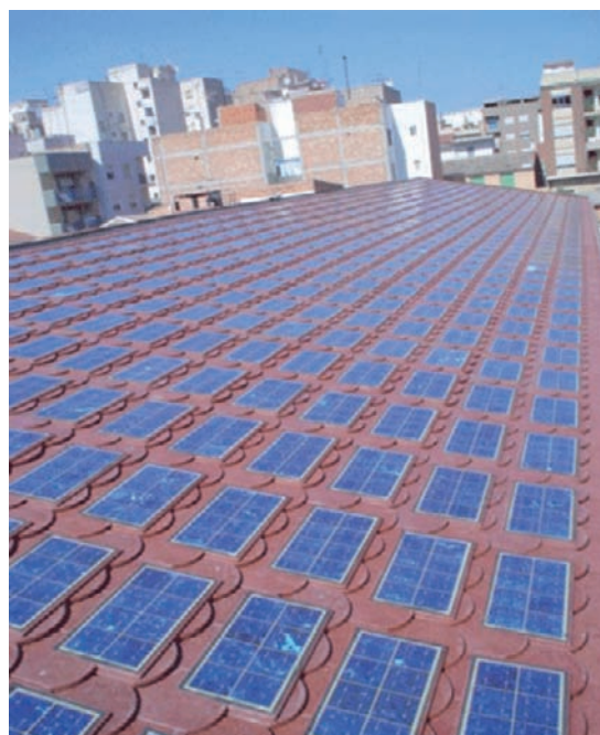
Crystalline silicon PV tiles integrated with a traditional roof.
