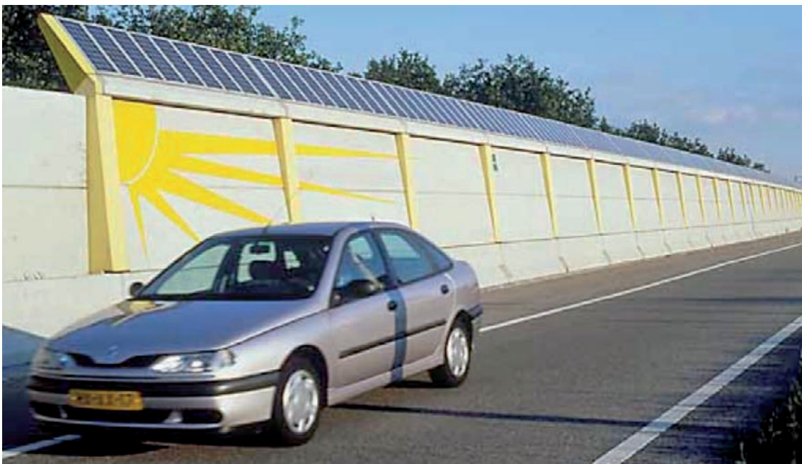
PV Noise Barrier A27 De Bilt, Utrecht - NETHERLANDS
