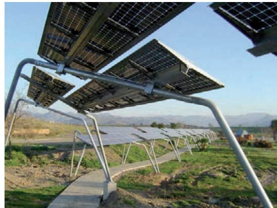
PV Pergola in the Andalusia Technology Park
