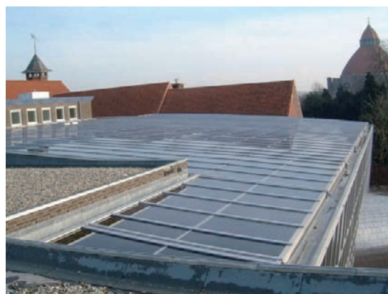
Flat roof in Dongen. Source: Scheuten Solar
