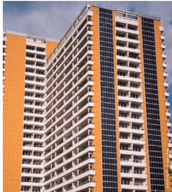
Façade integration in social housing residential building. Example of refurbishment. Berlin (Germany).. Source: PREDAC 5FP
