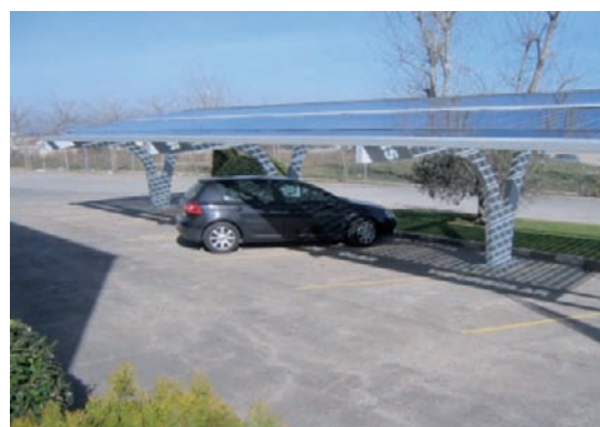
Car park in Manresa. Barcelona - Spain. Source: VIDURSOLAR
