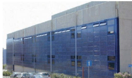
Integration of PV in the building of the Chemical Engineering Dept, National Technical University of Athens (by Germanos)
