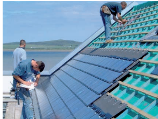
Installation of Modules in inclined roof.
